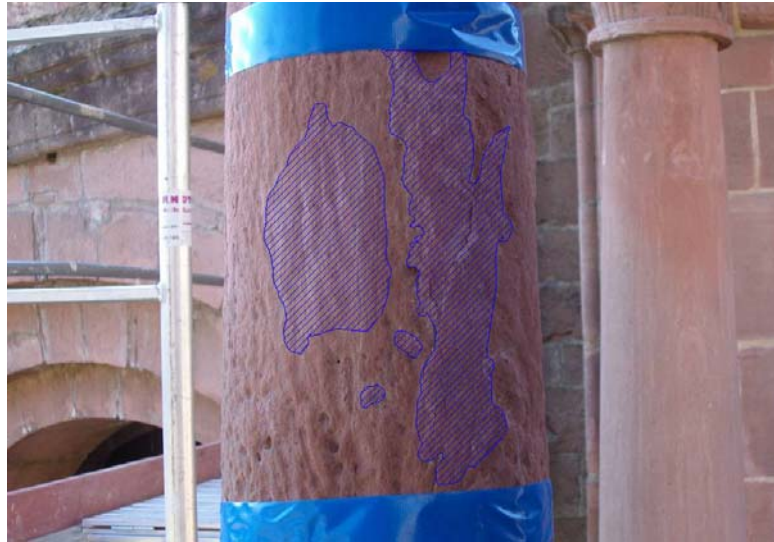
Figure 7: Results of IRT mapping drawn into the photograph.
